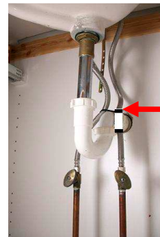
Install self-piercing needle valve on cold water line
